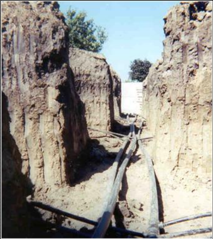
Trench Showing Header Piping
