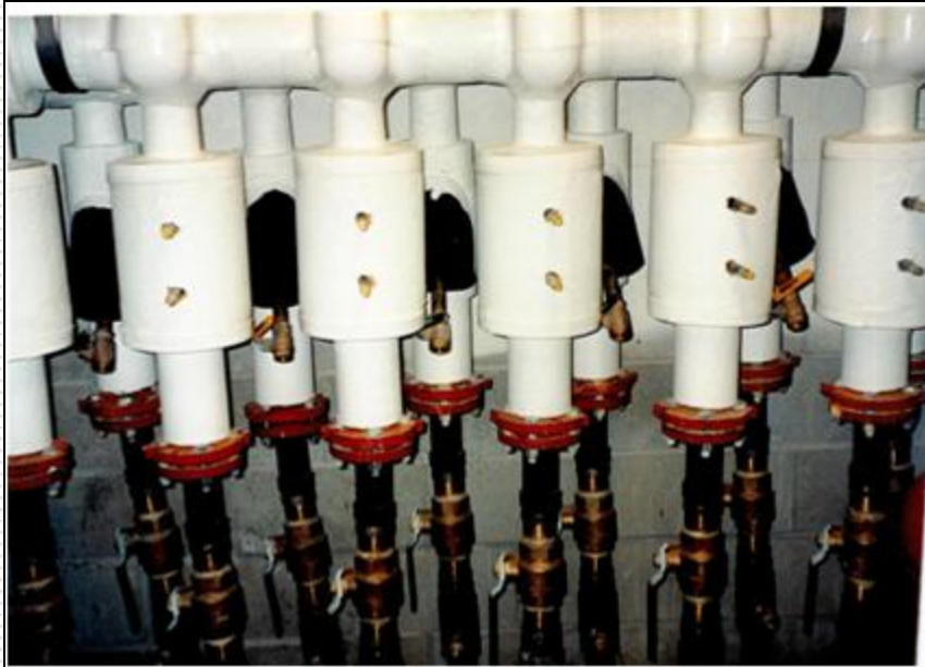
Header Manifold
