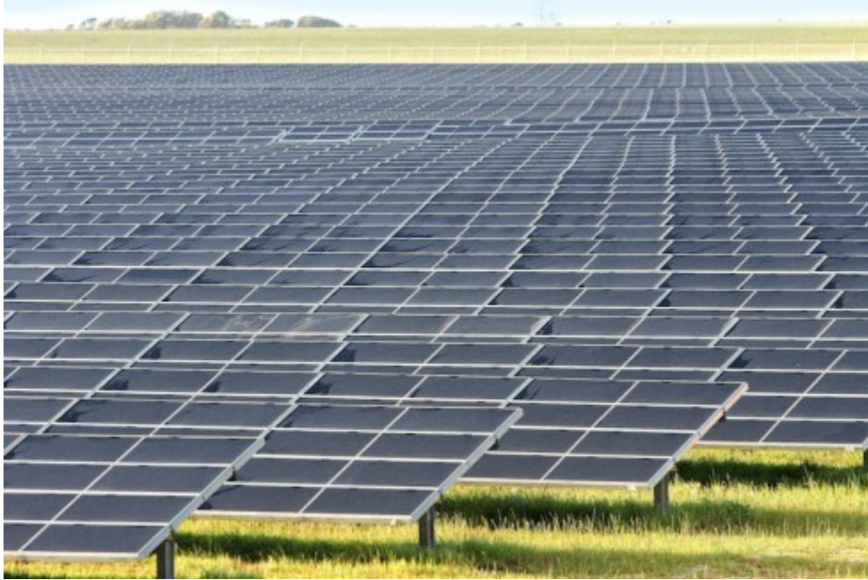
Figure 1: It takes 20-30 solar modules to generate the energy for one home for one year. This solar farm has about 400 modules per acre, enough to run 13 to 20 homes per acre.
