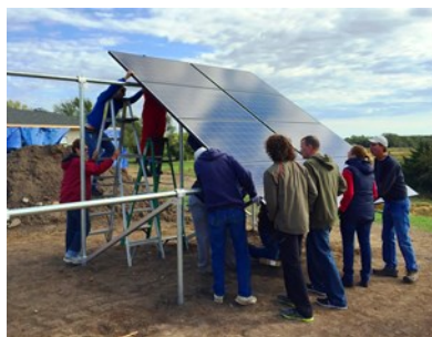
Photos from our Sept 2015 hands-on workshop installing a 6.24 kW Solar PV array
