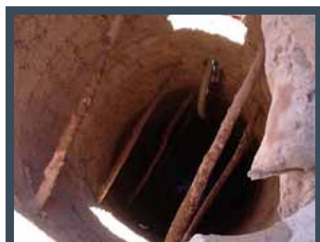
Illustration 17: Internal access to well (Bob Rout photograph)
