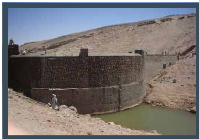
Illustration 13: Dam under construction
