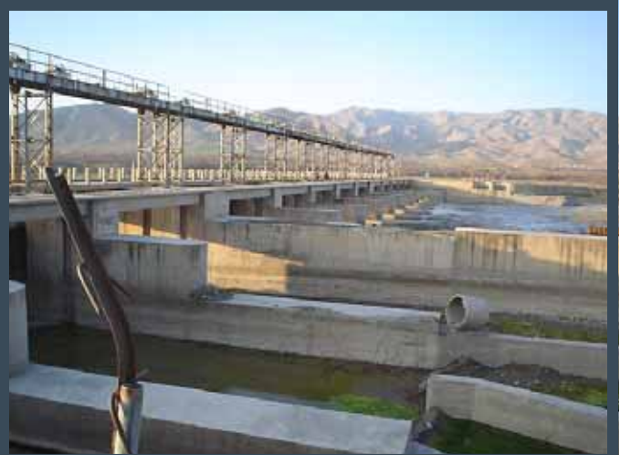
Illustration 21: Diversion weir, Kunduz-Khanabad (Bob Rout photograph)
