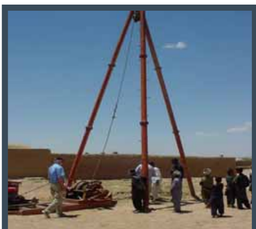
Illustration 19: Modern well-drilling (Bob Rout photograph)
