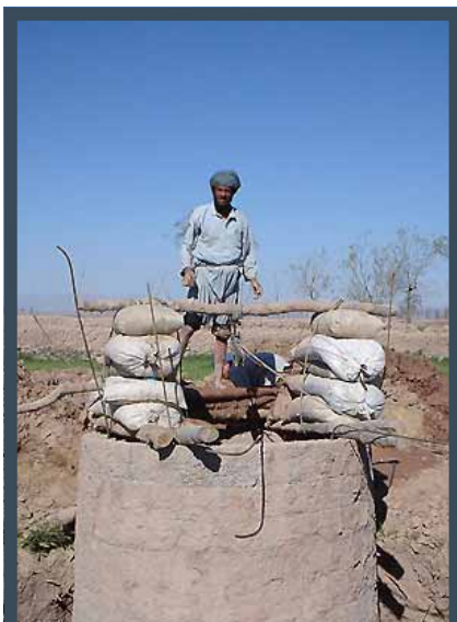
Illustration 18: Well construction traditional method (Bob Rout photograph)
