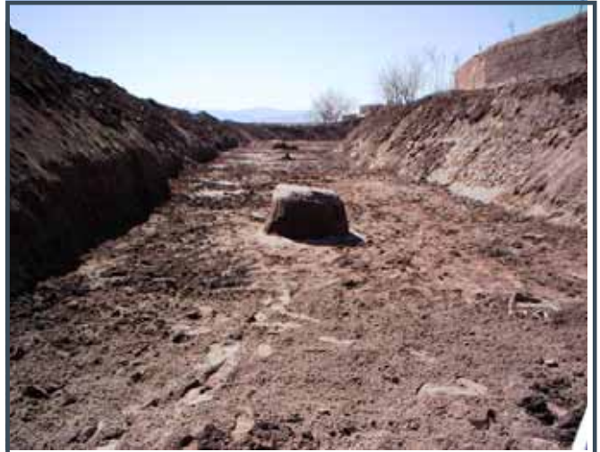
Illustration 3: Main canal after de-silting
